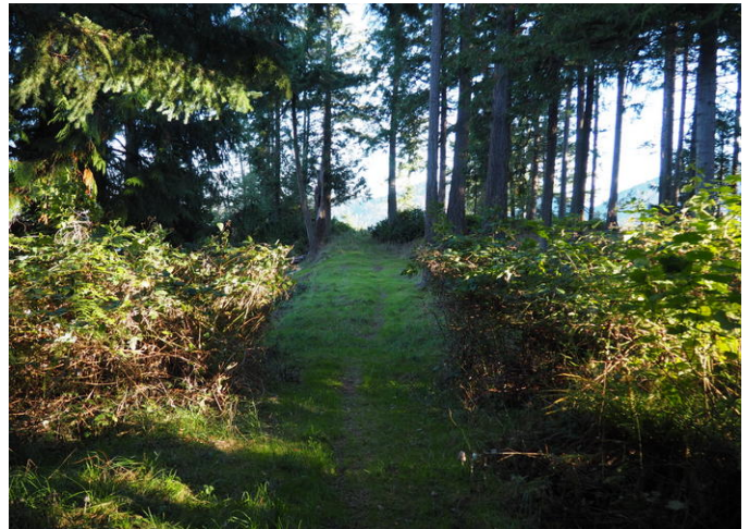
Roughed in driveway leads to one of the building sites.
