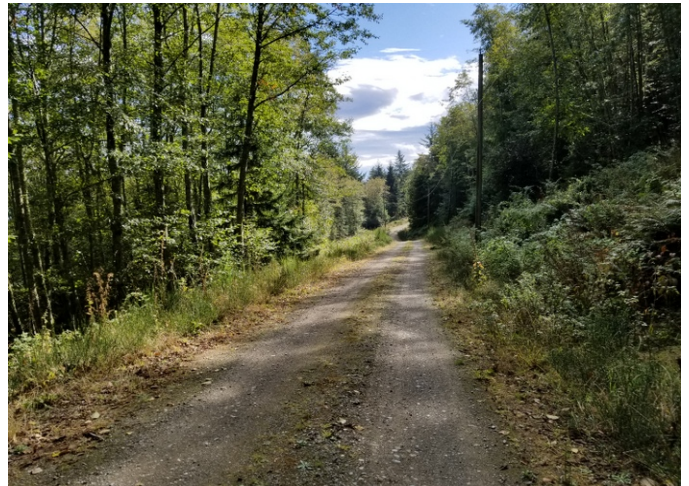
Beau Vista Lane. Power runs along this private easement.
