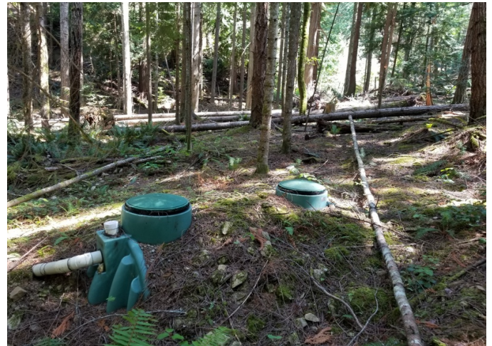
Septic system has been installed.
