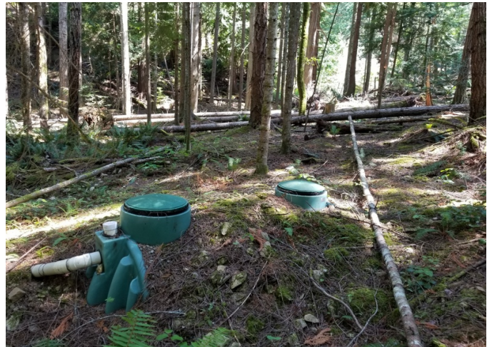
Septic system has been installed.
