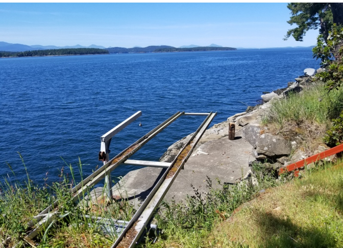
Boat launch and lift. View to the west and northwest. Short stair case down to the cemented pad.
